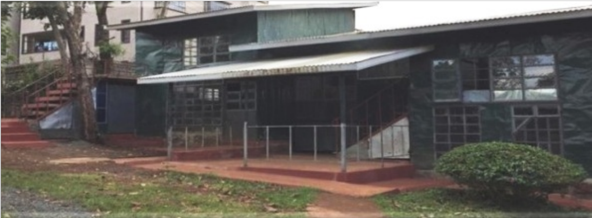
The newly constructed addition for CAL at the APMI school in Ngong
